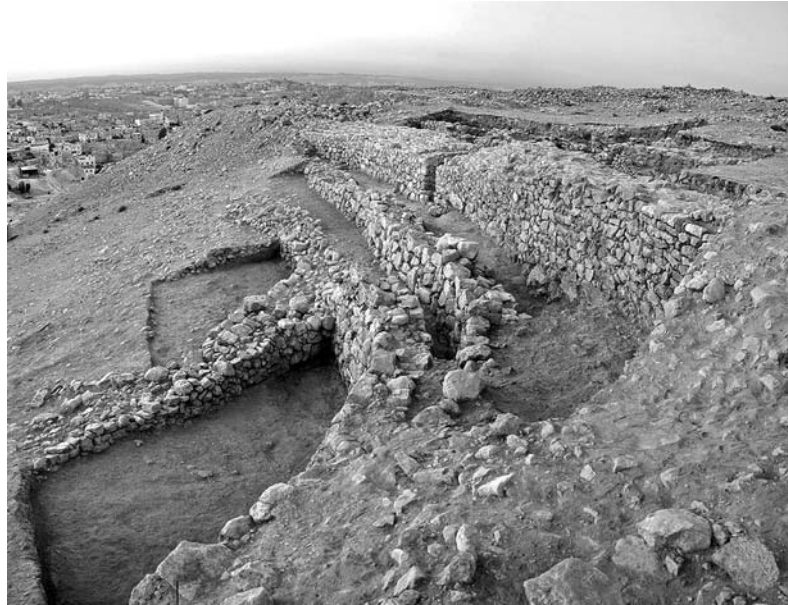
Figure 10. Khirbet al-Batrawy: the EB IIIB (2500-2300 BC) triple line of fortifications, from west: to the left, EB IIIB Scarp-Wall W.165 with protruding wall W.177; in the middle, EB IIIA-B Outer Wall W.155, gradually turning northwards; to the right, the EB II-III Main City-Wall.
